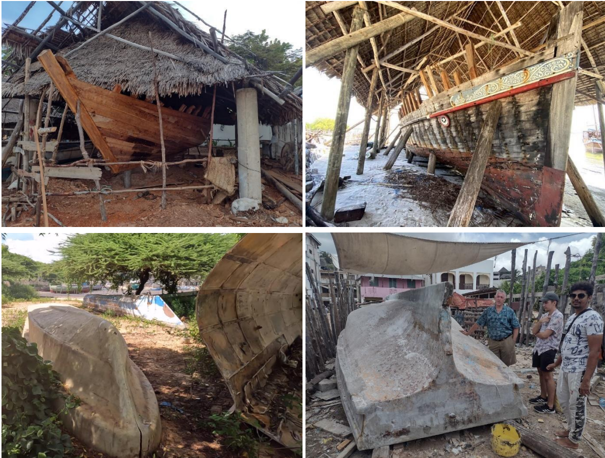
Figure 7: Construction Methods. A new wooden build (top left), an older dhow, Utamaduni, prior to renewal (top right), fibreglass taxiboat moulds (bottom left), “Almas” – a fibreglass dhow under construction (bottom right)
