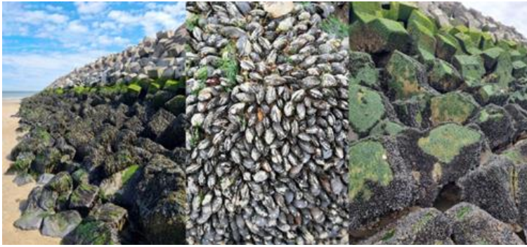
Figure 4 – Xblocs in the North Sea with marine growth
