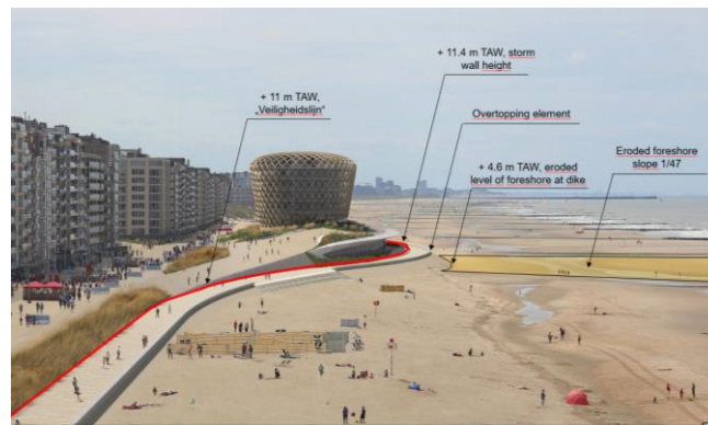
Figure 2. CASINO stilling wave basin in Middelkerke, Belgium (Adapted based on source: Witteveen + Bos)
