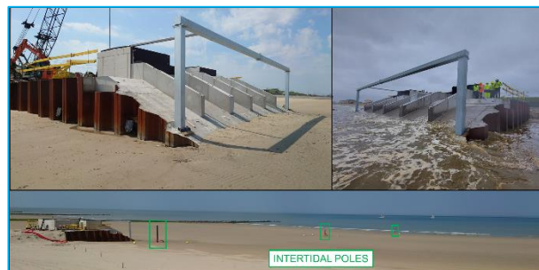
Figure 2. The research dike and intertidal poles at low tide (top left and bottom) and high tide (top right).
