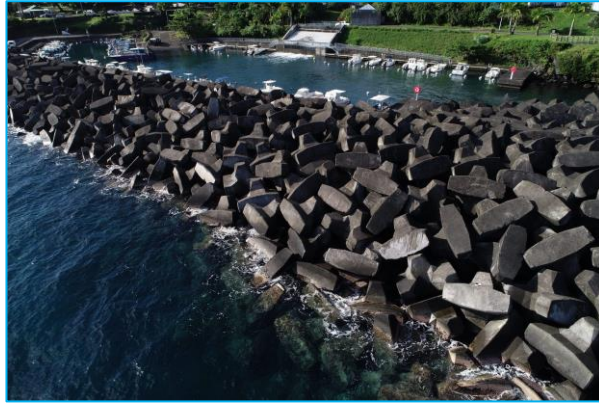
Figure 1. ACCROPODE™ I breakwater of Sainte-Rose harbour, La Réunion.
