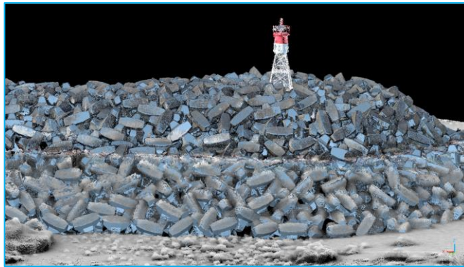
Figure 2. Survey point cloud and 3D model of Sainte-Rose breakwater roundhead.
