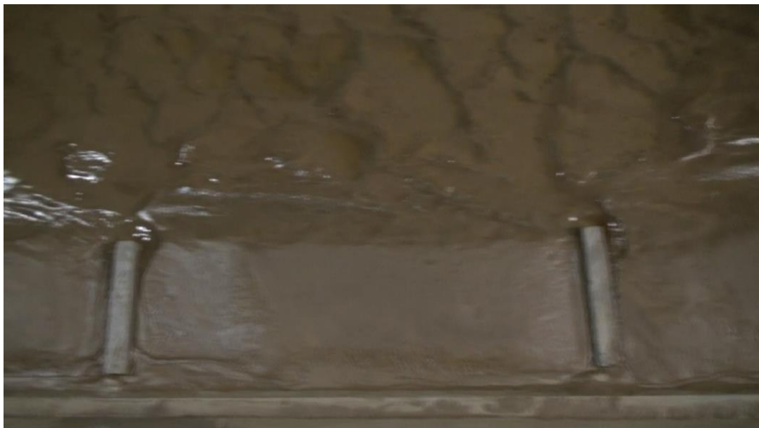
Figure 11. Photo of the beach near the seawall after the construction of spur dikes.
