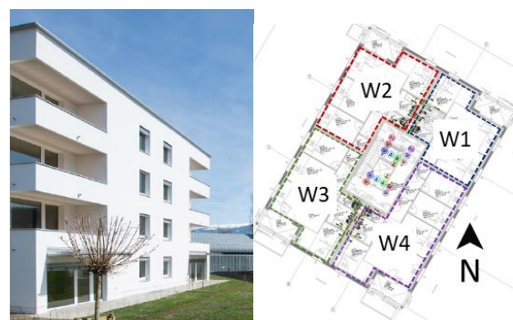
Fig. 2 – Outside view of the multi-family building and a floor plan (NHT, Innsbruck).
