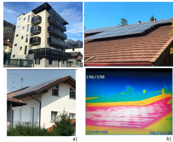
Fig.1. a) Examples of rooftop PV systems in existing buildings in Northern Italy with a) showing solar array shading of apartment roof complex. b) Visible and IR image illustrating impact of shading from photovoltaics on thermal heat gain. Colour is proportional to temperature: white/ red hottest, and black and blue coolest.
