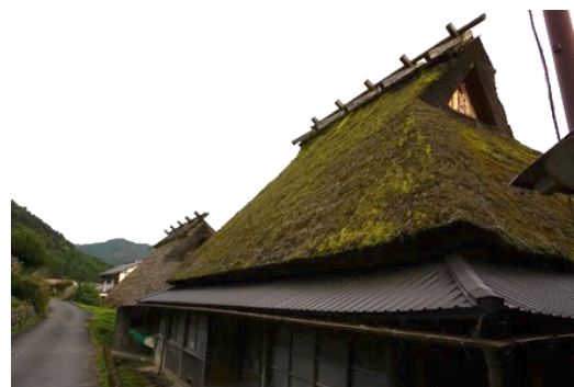
Fig. 1- Traditional Japanese house with a thatched roof. In summer, windows and partitions are opened, and in winter, windows are closed with the use of a wood stove.
