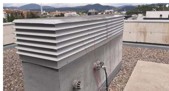
Fig. 5. - Taking measurements in AC Building.
