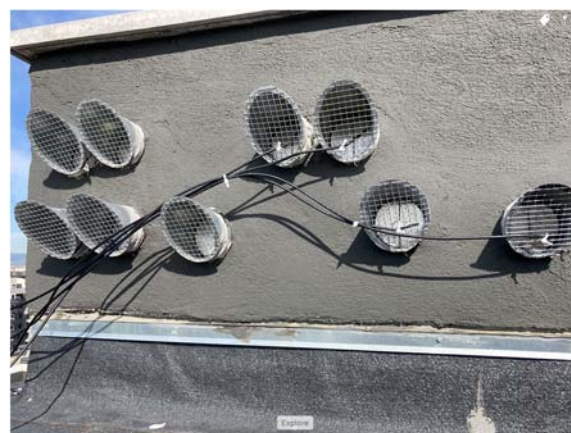
Fig. 4. - Taking measurements in AB Building.
