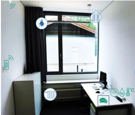
Fig. 2 – A room with indoor climate monitoring devices
