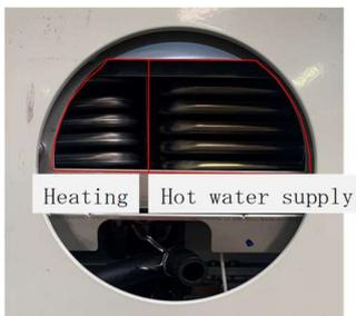
Figure8.internal shape of the exhaust outlet
