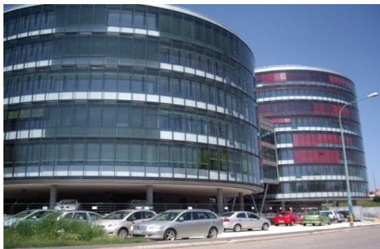
Fig. 10- View of office building B
