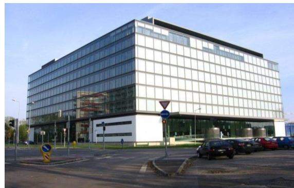
Fig. 8- View of office building A
