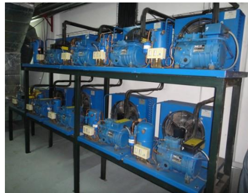
Fig. 2- Refrigerating Condensers
