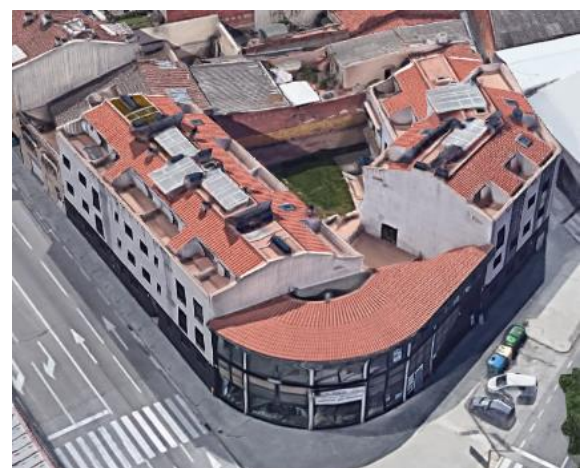
Fig. 3 – Terrassa building demo site, aerial view
