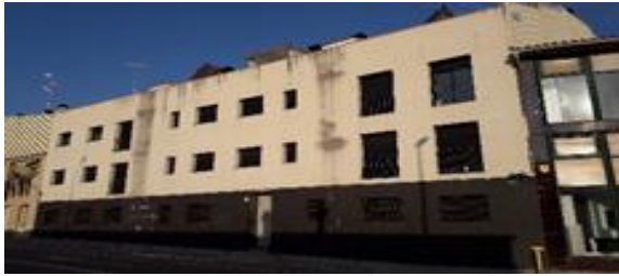
Fig. 4 – Terrassa building demo site, east façade
