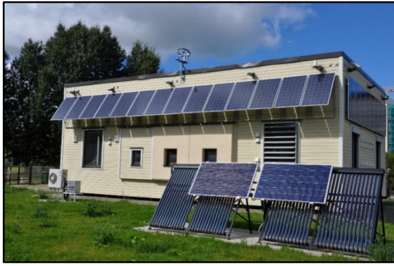
Fig. 1 – Tallinn University of Technology nZEB test facility
