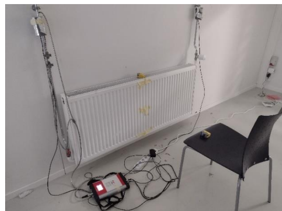
Fig. 2 – Radiator, TinyTag data loggers and flow meter
