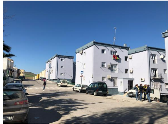
Fig. 11- Current state of the district
