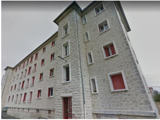
Fig. 3 - Real building studied before rehabilitation.
