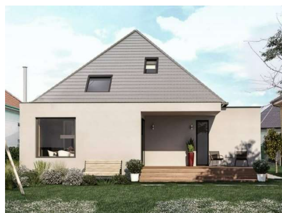
Fig. 6 – View of the family house from the garden after renovation [2, 3, 4].
