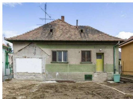
Fig. 5 – View of the family house from the garden before renovation [2, 3, 4].
