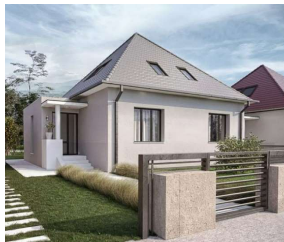
Fig. 4 – State of the house after renovation [2, 3, 4].
