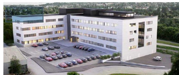
Fig. 1 - Body of this office building.
