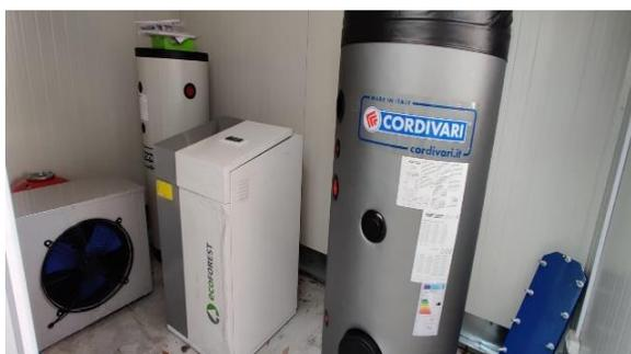
**Fig. 5** – Heat pump used within the proposed system
